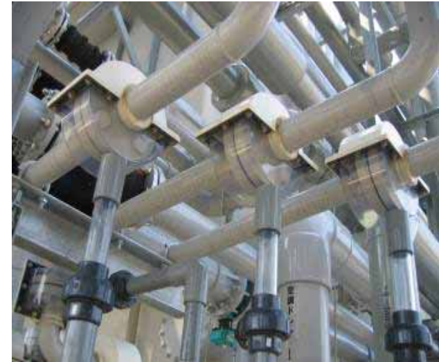
[配管の継手部二重化]
